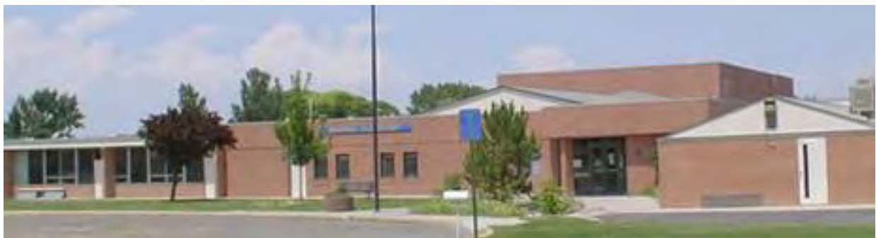
One of 79 MCVSD buildings receiving energy-efficient lighting upgrades.
