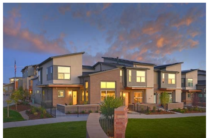
Top: Chandler at Little Cottonwood Canyon by Garbett Construction, Salt Lake City, UT; Bottom: Courtyard Rows by Thrive Home Builders, Denver, CO; Photos courtesy U.S. DOE
