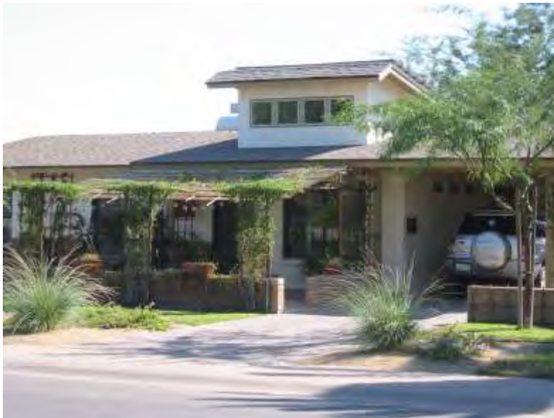
Shaded Entry Courtyard
